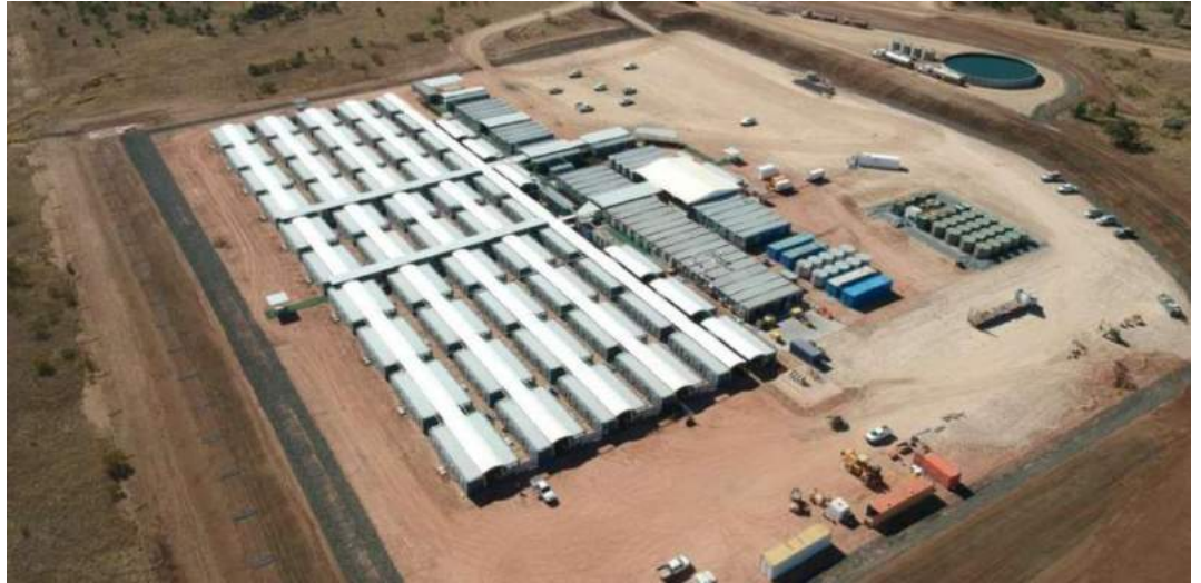
Example of accommodation camp
